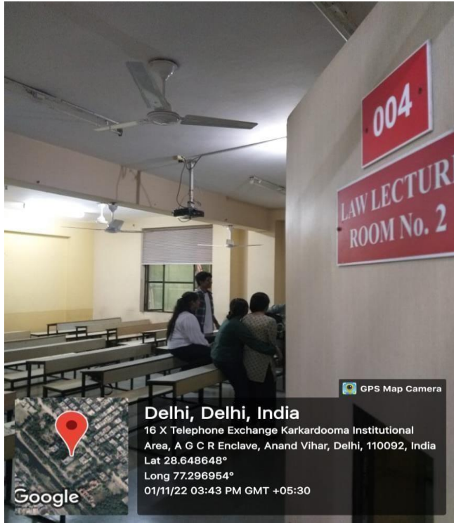
ROOM NO-004, WALL MOUNTED PROJECTOR
